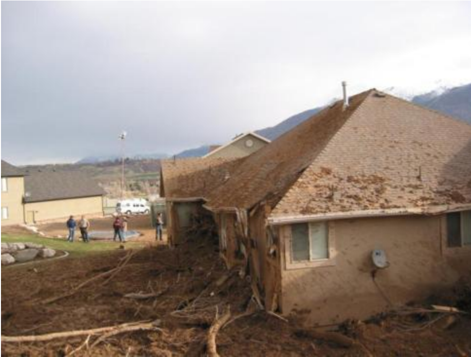
Weber County Landslide 2006
